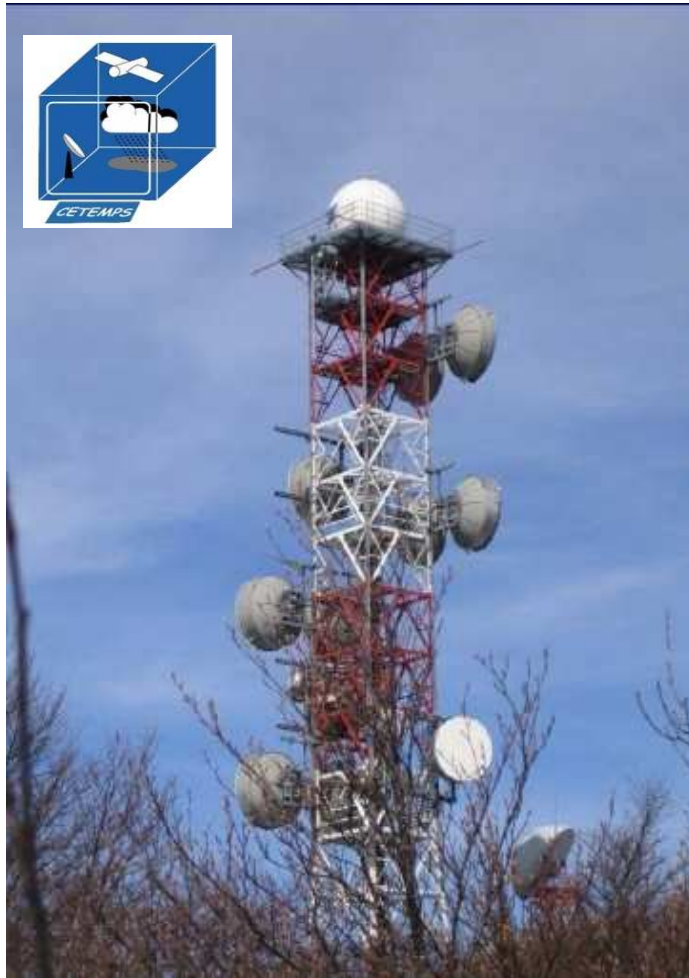
PYLON OF 50 METERS IN MONTE MIDIA
